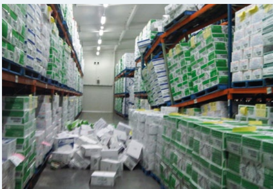
Damage to cool-store racking following the earthquake on 22 February
