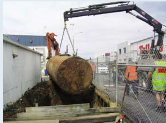
Removal of the old diesel tank
