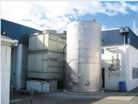
New water storage tank
