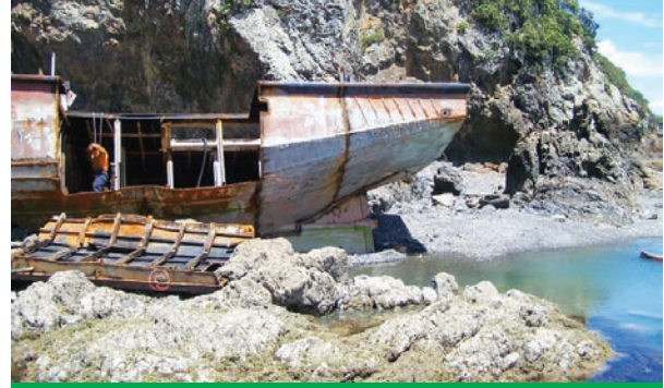
San Cuvier being dismantled
