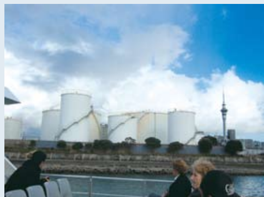
Tank Farm as seen from the harbour
