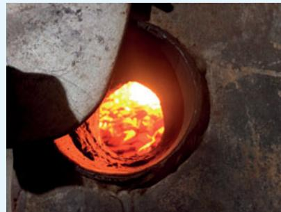
**Photo:** Wood chip alight in our fishmeal plant boiler
