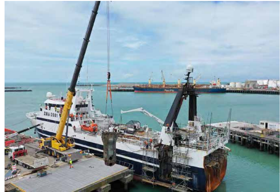
ABOVE Sanford deepwater vessel the San Discovery, boiler replacement.
