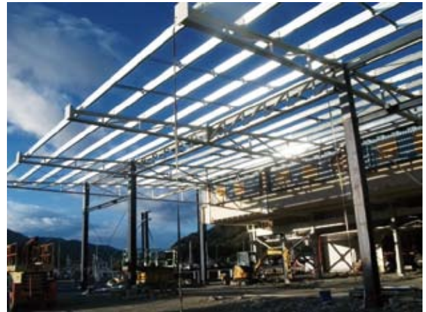
Roof extension underway during the Havelock plant upgrade
