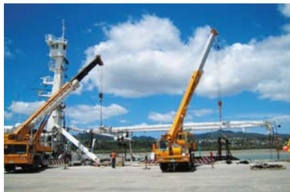
San Nanumea – main boom being removed from vessel for repair
