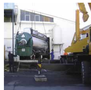
Installing new fishmeal drier, Timaru
