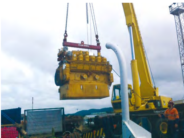
San Nikunau – new starboard generator being lifted onto vessel for installation
